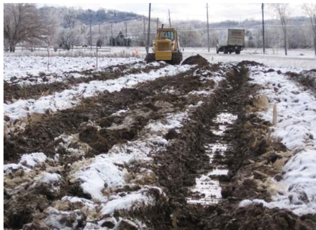
Working in the trenches.
