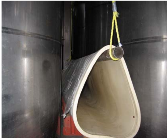
#1: Spare bladder hanging between tanks, just in case!
